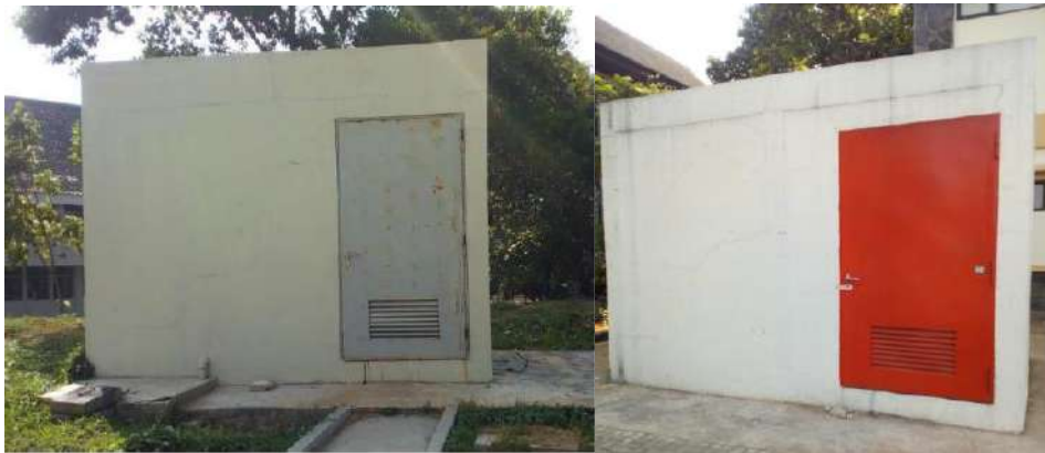
Figure 46. Hazardous Waste Treatment Facility
