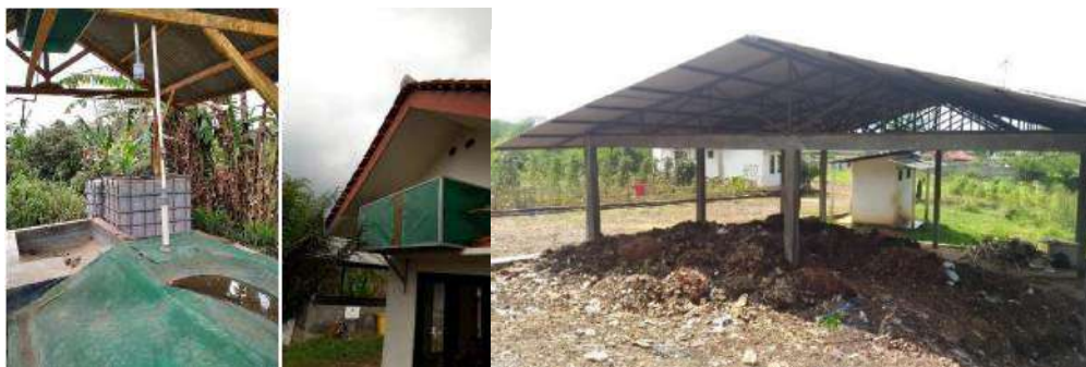
Figure 13. Biogas Technology Management and Compost House as Waste Management
