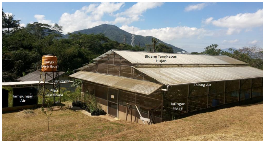
Figure 10. Rainwater Harvesting System at the ALG Greenhouse FTIP
