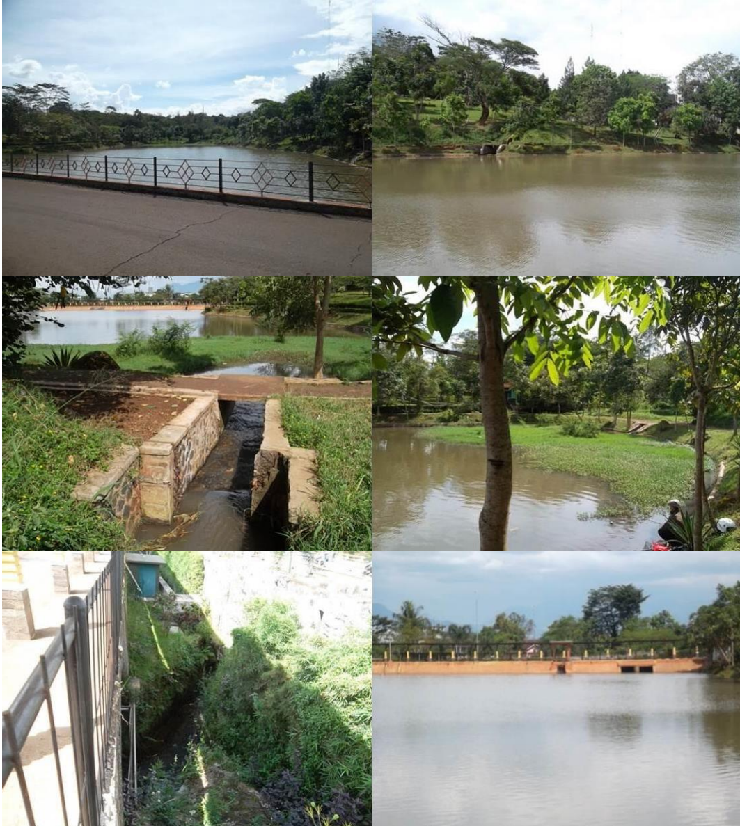
Drainage at the western side of UNPAD Campus (Arboretum Check Dam) dammed to reduce the water runoff coefficient
