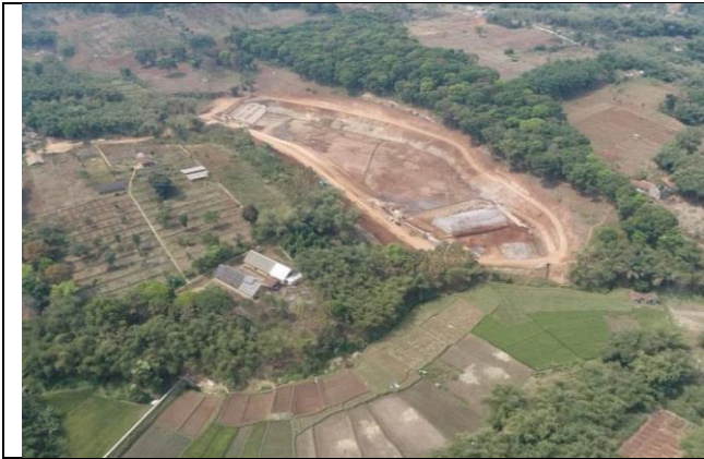
Retention ponds area
