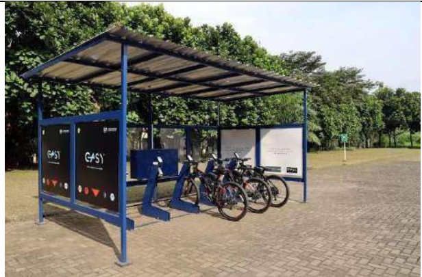
Solar electric bicycle shelter
