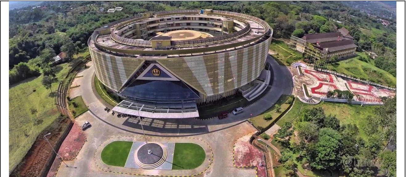
Natural Ventilation system
