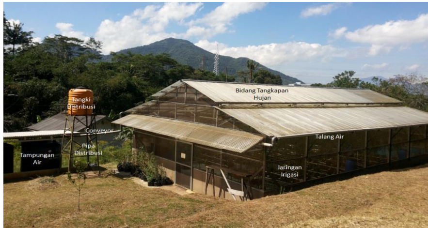
Rainwater Harvesting System at the ALG Greenhouse FTIP
