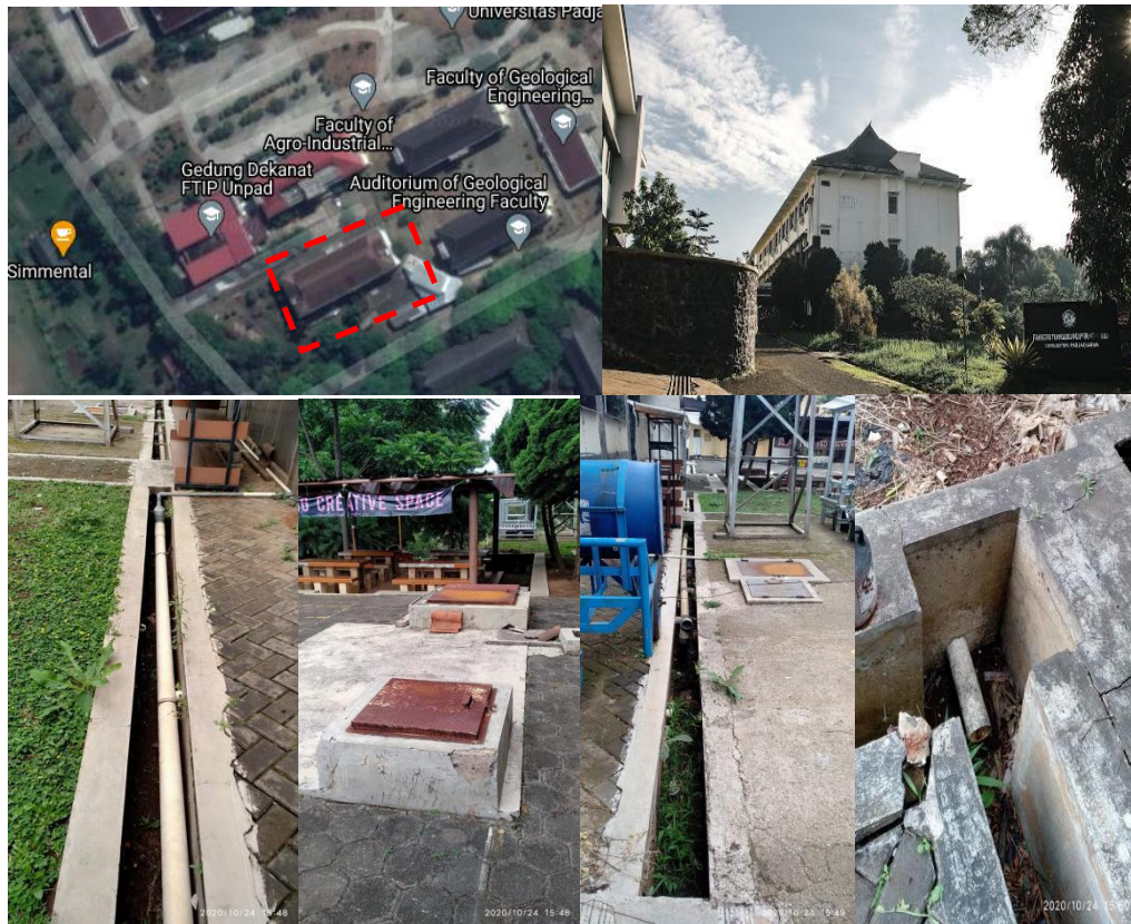
Rainwater harvesting system at the TPB FTIP building
