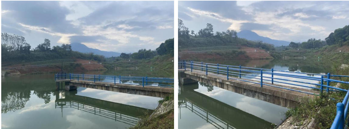
UNPAD Basin (After being flooded)
