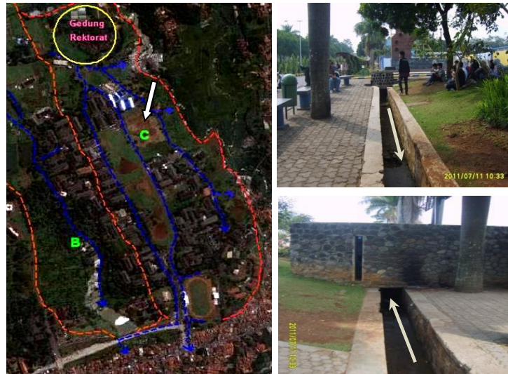
Drainage System of Unpad Jatiningor Central Campus
