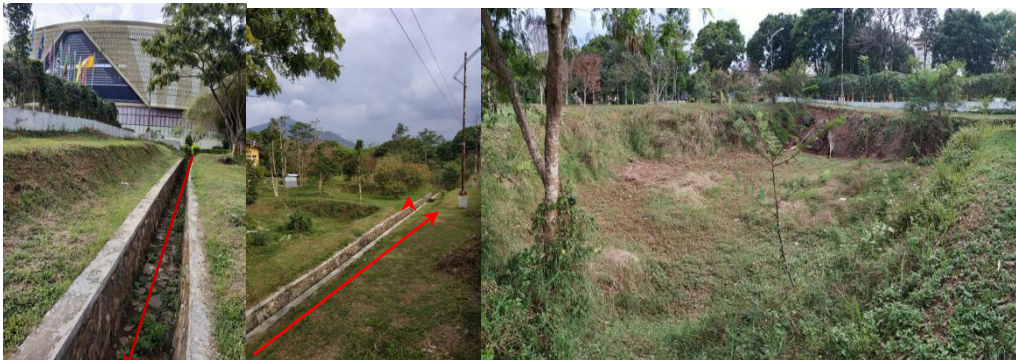
Rectorate Rain Garden functions to accommodate and absorb surface runoff from the rectorate building
