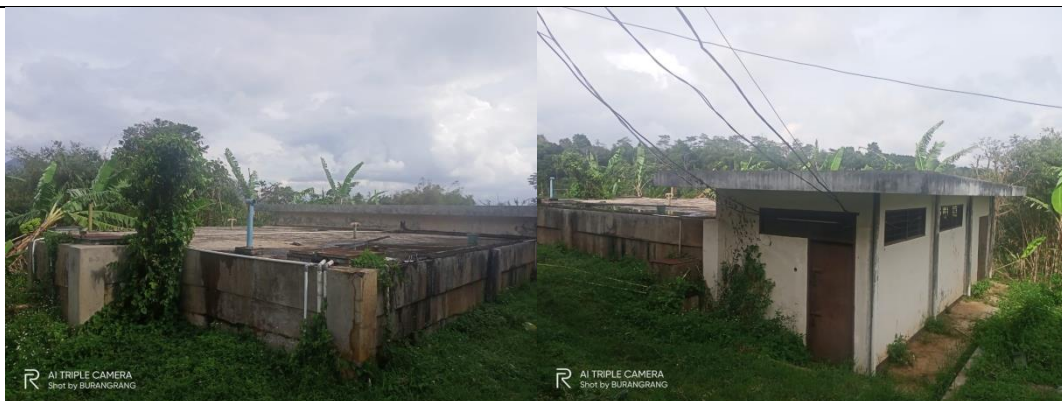
Main water reservoir 2
