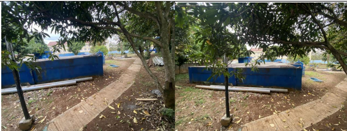
Main water reservoir
