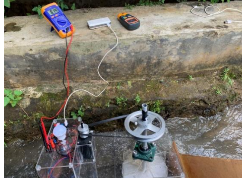
Portable Nano Hydro Generator Monitoring
