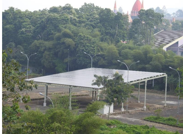
Solar Panel in Parking lot
