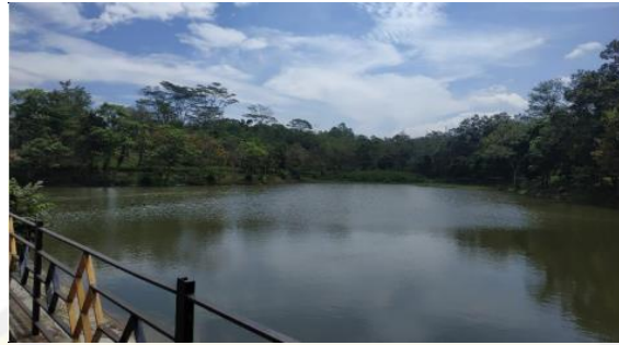
The drainage system that empties into the checkdam of Universitas Padjadjaran
