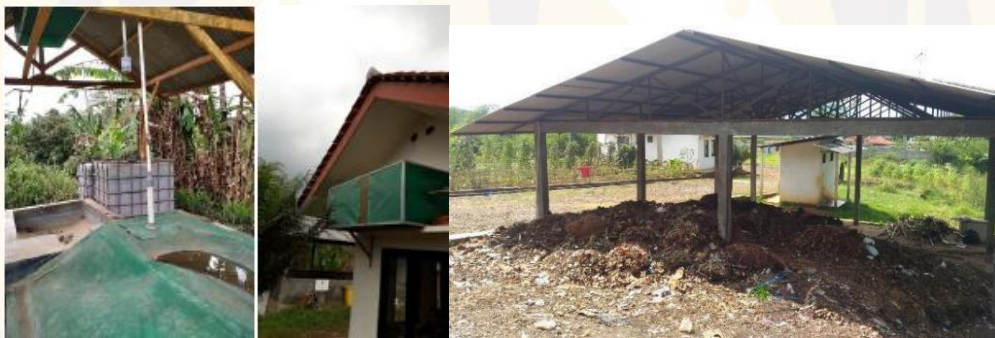
Figure 13. Management of Biogas Technology and Compost Houses in Waste Management
