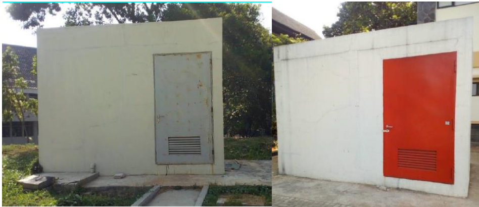
Figure 52. Hazardous Waste Processing Facilities
