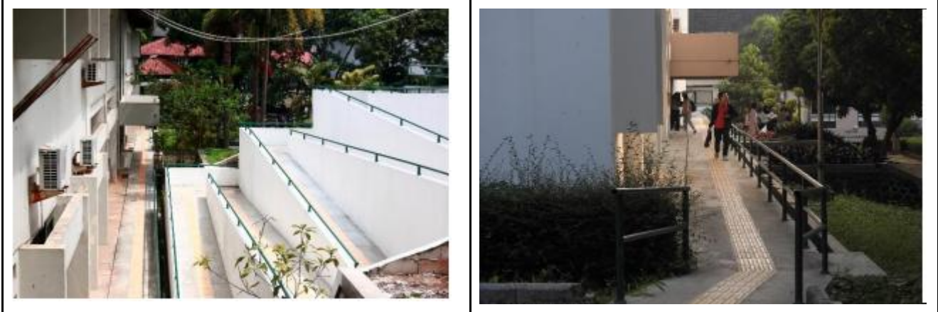
Examples of ramps with guiding blocks for pedestrians at Universitas Padjadjaran.
