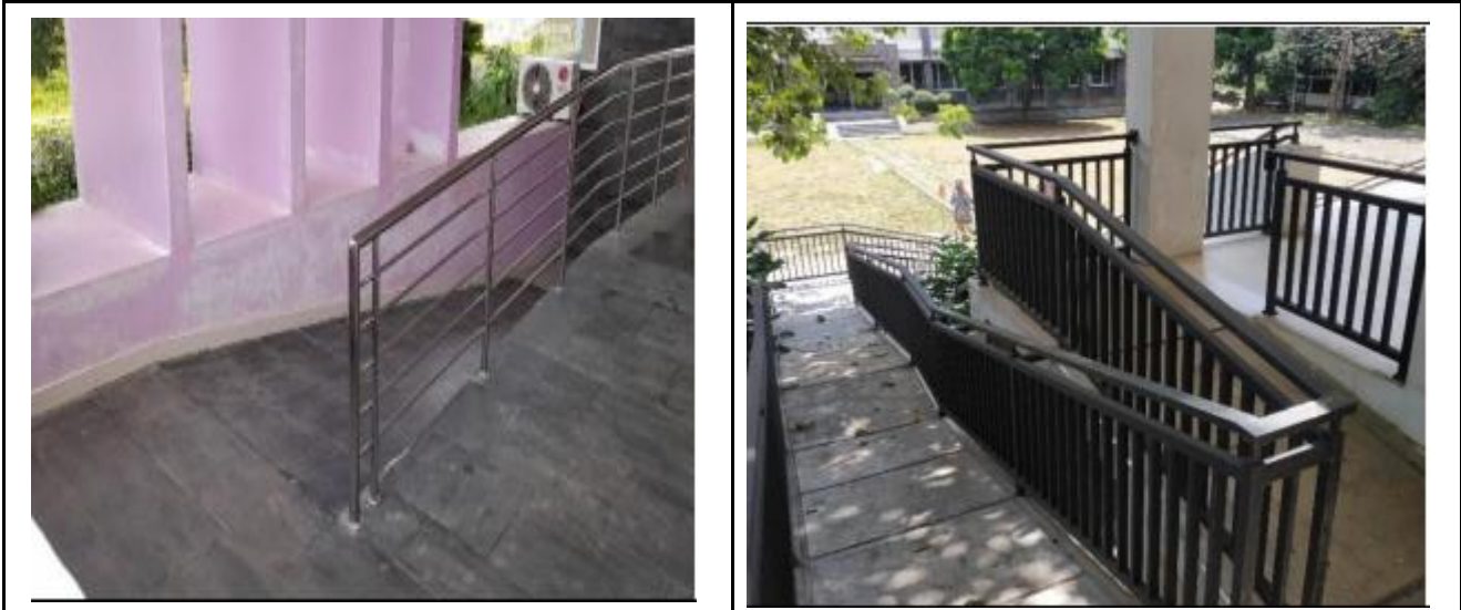
Examples of ramp facilities at Universitas Padjadjaran.
